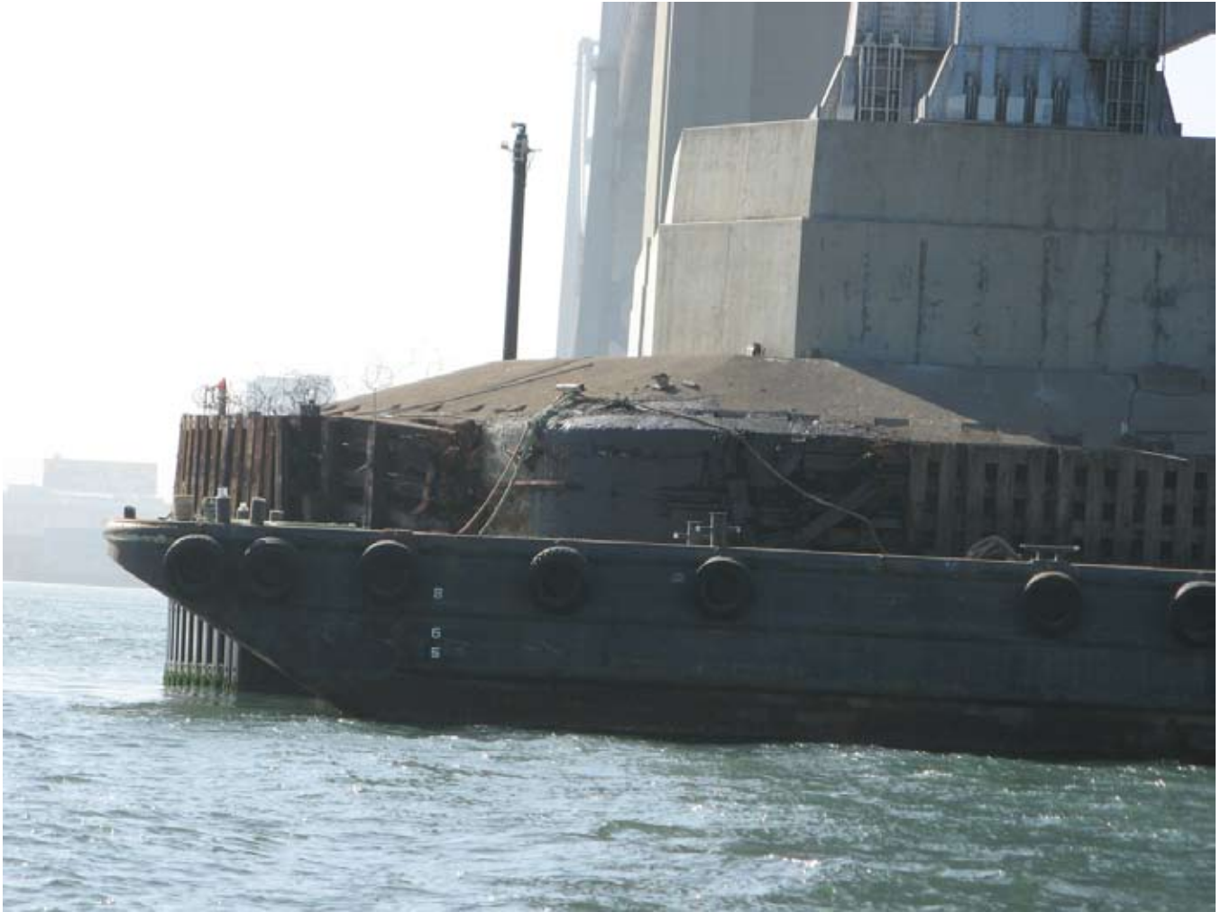
Oil still stained the Bay Bridge Pier where the Cosco Busan hit more than a week later
